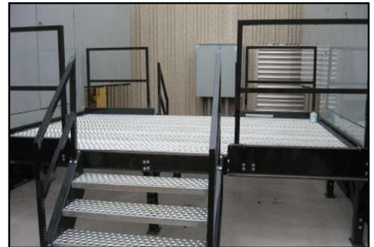
*Staircase and platform installed between two gen-sets.*
